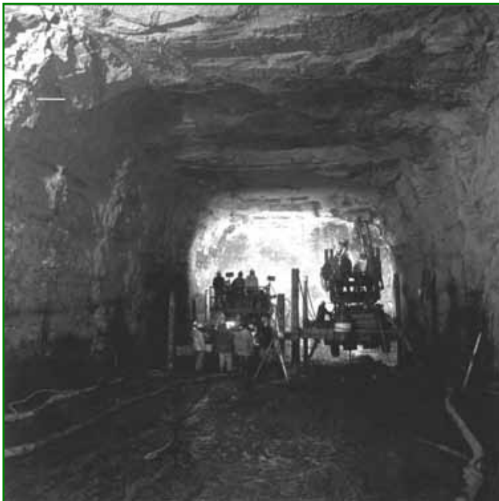
Figure 7-19 – Wesleyville Access Tunnel
