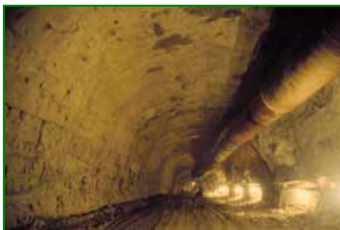
Figure 7-22 – Darlington Tunnel Top Heading Excavation
