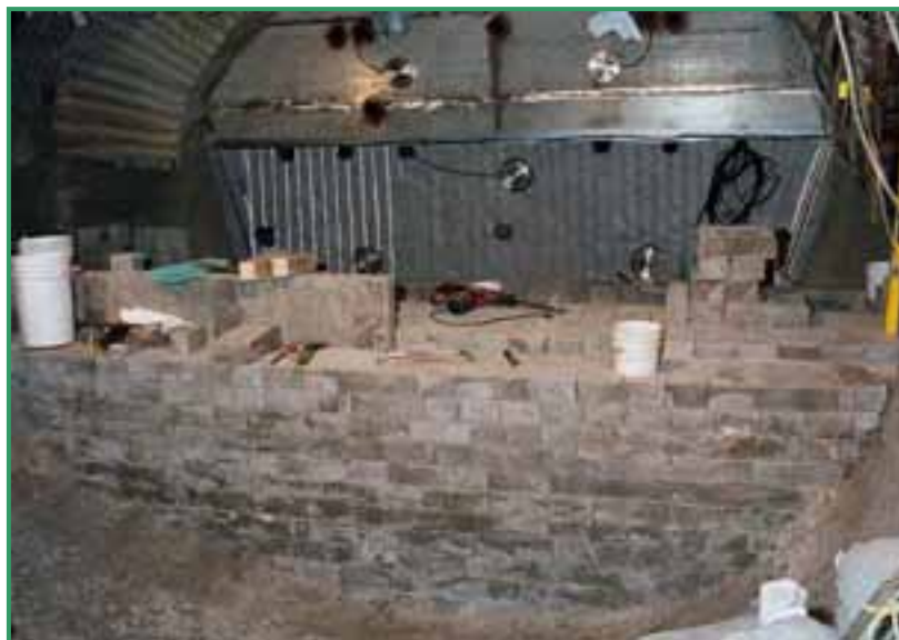
Figure 14-4 – Example of pre-compacted bentonite blocks [R102]
